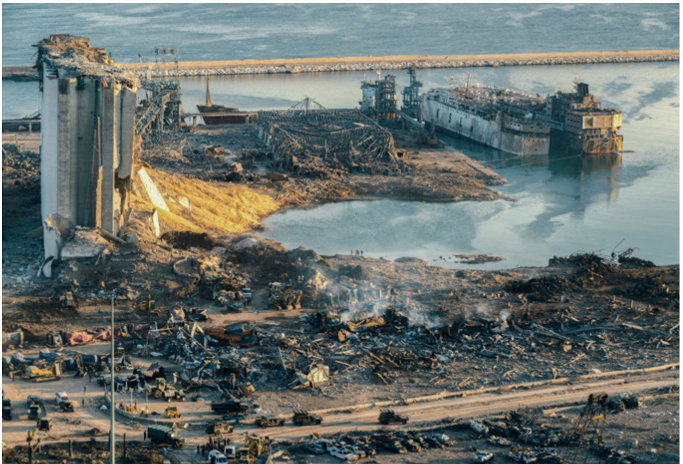
Picture 2: aftermath of Beirut's port ammonium nitrate explosion incident (estimated 2,750 metric tonnes) in 2020
